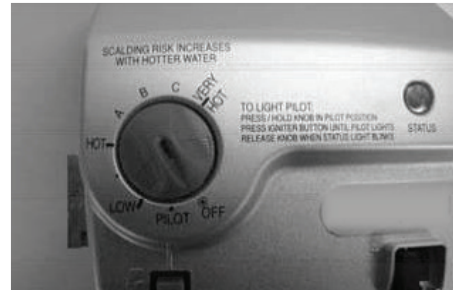
Rotate knob counter-clockwise to the "OFF" position
