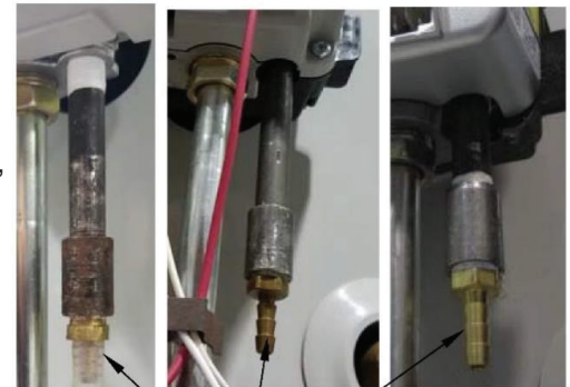
Pressure tap shown installed
